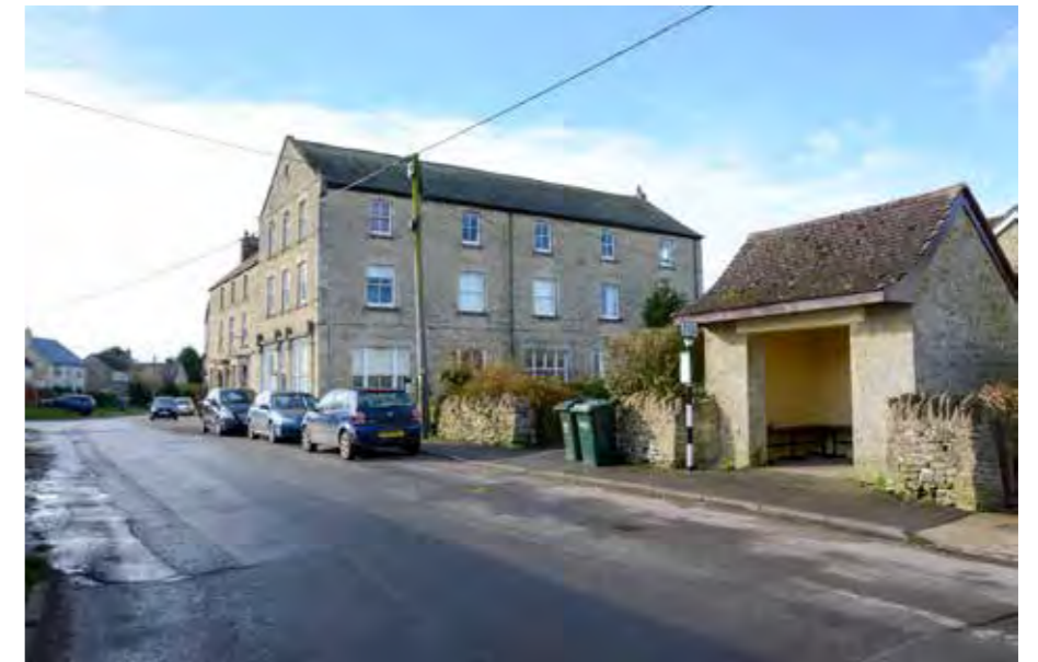
A. 28 East Street (Old Dew's Shop)
