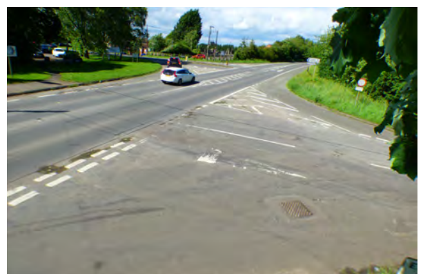
Excessive junction geometry extends the highway into Ardley's centre
