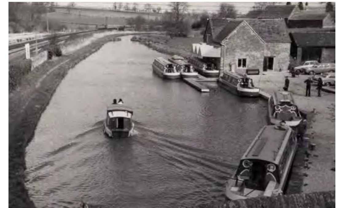
Lower Heyford: Oxford Canal from bridge
