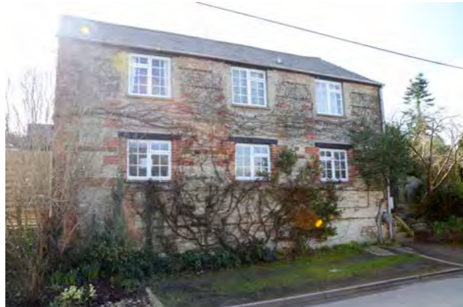
Limestone, marlstone and red brick can regularly be found complimenting each other in the facades
