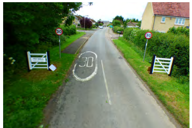
The entry to Fretwell is clearer, with markings gone and widths reduced
