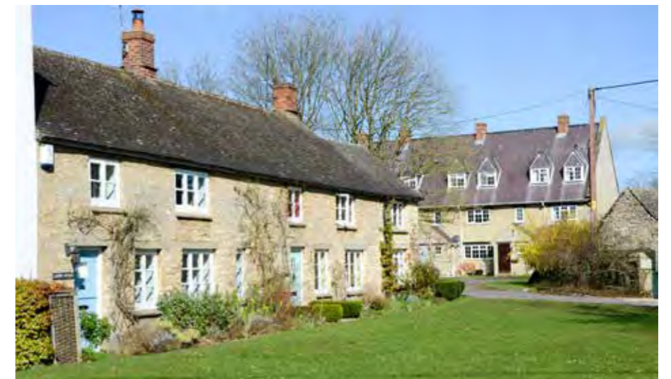
More recent development (rear) has favoured dormer third storeys which are out of scale with the historic development within the village (fore)
