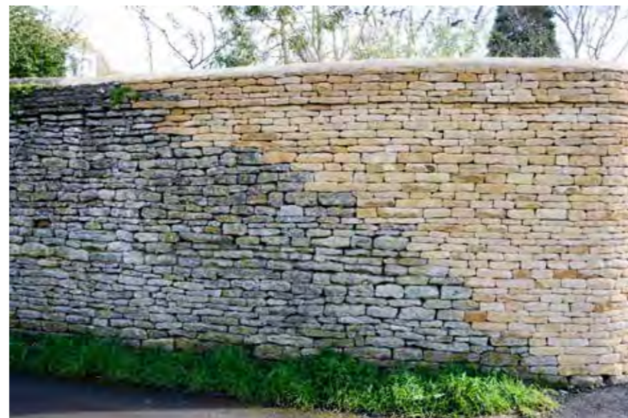
High quality sympathetic repairs to stone walls protect the character of the village
