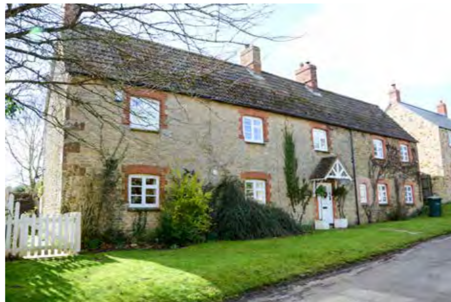
Vernacular housing of limestone with red brick detailing around timber windows
