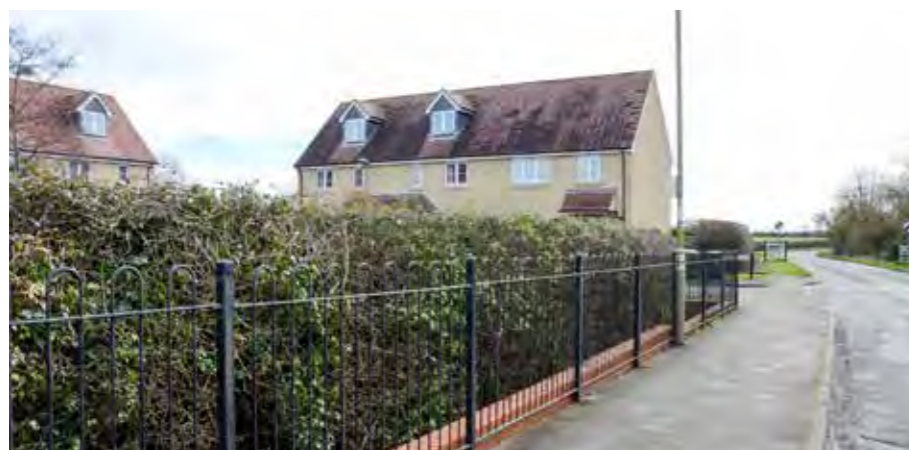
Recent bow top fencing out of character with the village
